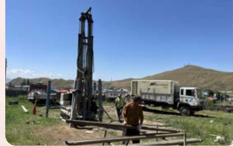
water well drilling (top) & masonry (bottom)
