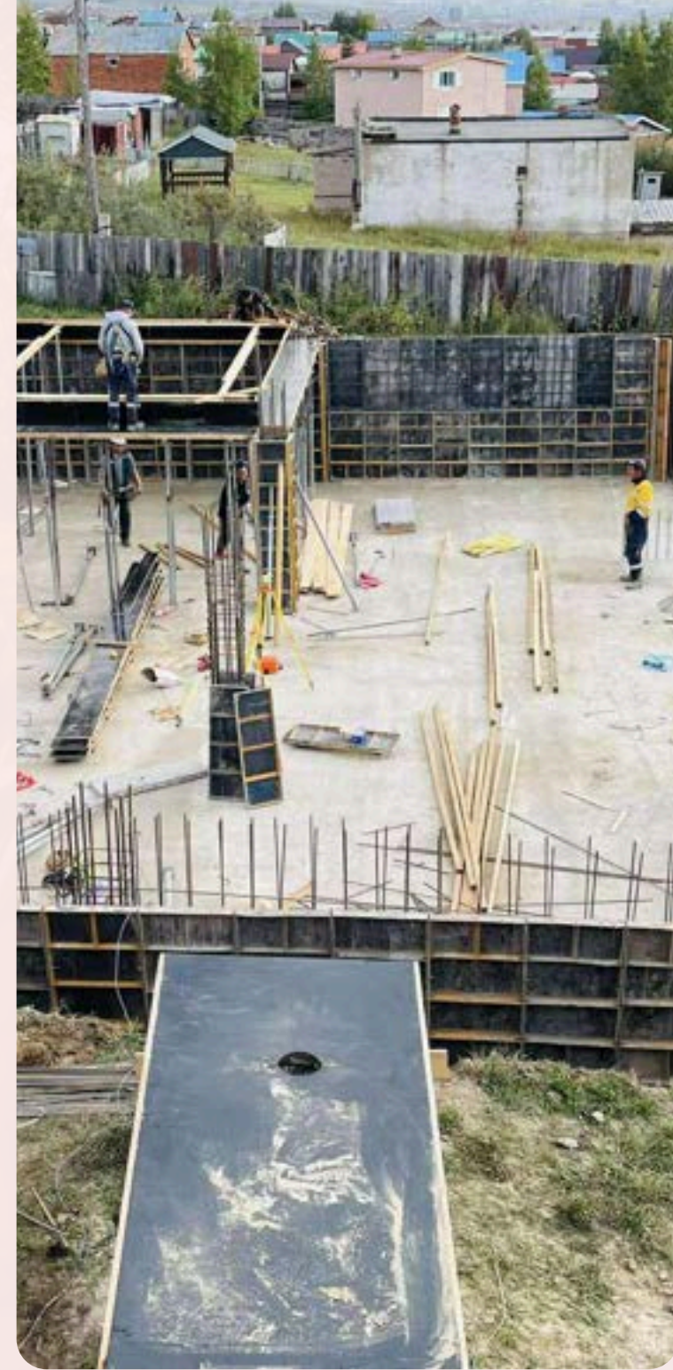
reinforced foundations
